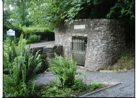
Bryan and Ray cleaning out the Wells in 2001 and the Wells today
